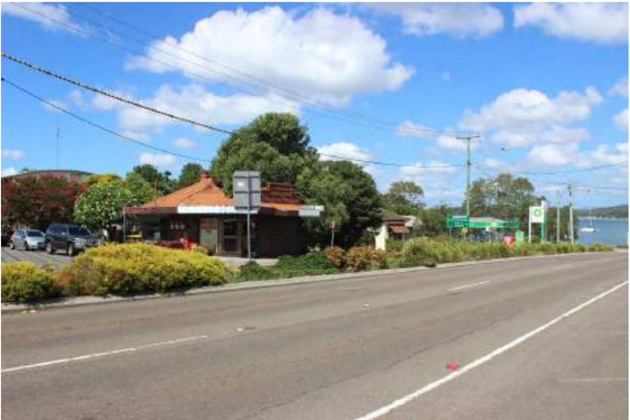
Photograph 1 - Existing Site Development – King Street
